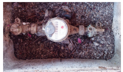
Figure 5-7: Water meter
