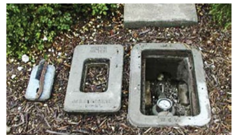
Figure 5-7: Water meter
