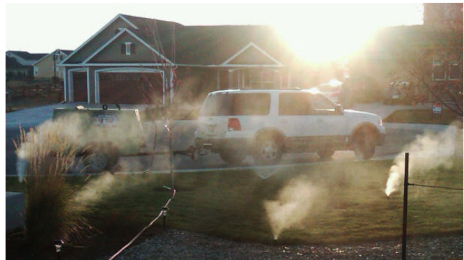
Figure 6-5: Blowing out one station at a time. (Peakview Irrigation)
