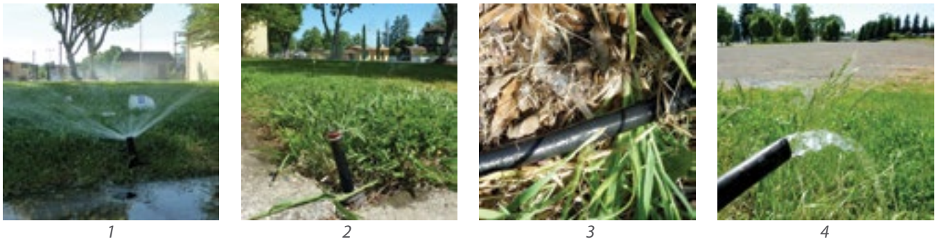
Figure 6-2: Left to right (1) (2) tilted sprinkler heads, (3) missing drip emitter, (4) severed drip line
