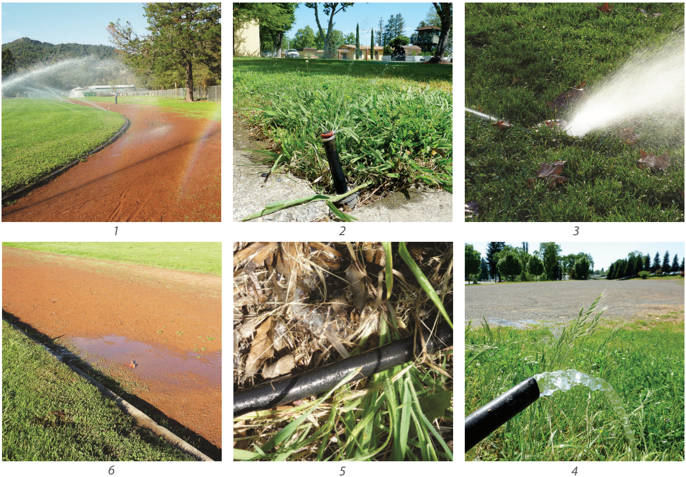
Figure 7-7: Clockwise (1) overspray, (2) tilted head, (3) head below grade, (4) severed drip line, (5) missing emitter, (6) leaking seals
